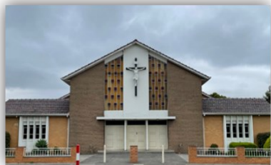
132 Melbourne Ave, Glenroy
